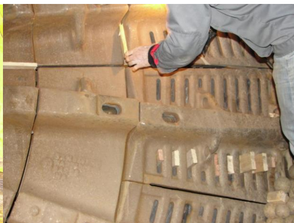
Figure 9 Installation of wooden wedges imitating lifters' operation
